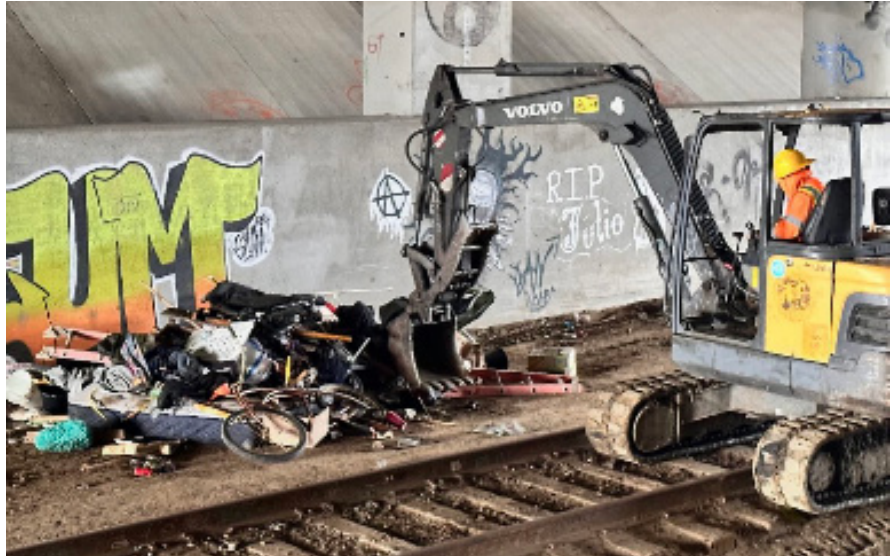
UNION PACIFIC crews helped clean up trash and debris (HBPD photo).
