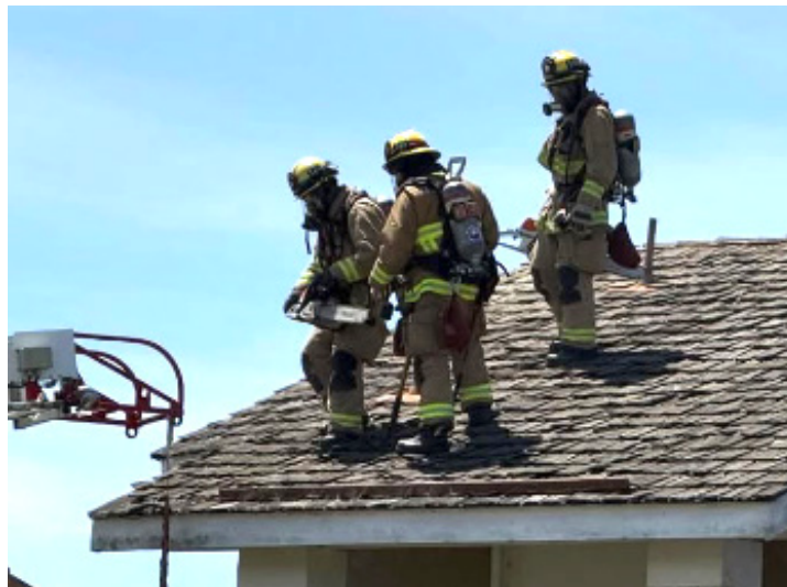
A bedroom fire on the second floor of a single-family home in the 6000 block of Moonfield Drive near Talbert Avenue in Huntington Beach was quickly knocked down by the Huntington Beach Fire Department on Wednesday, confining the blaze to the upper portion of the home. No injuries were reported (HBFD photo).
